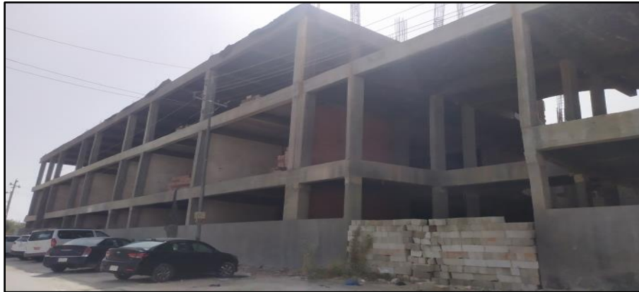
Image (14). Unfinished building on Street 40 Source: Field study dated 8-4-2022
